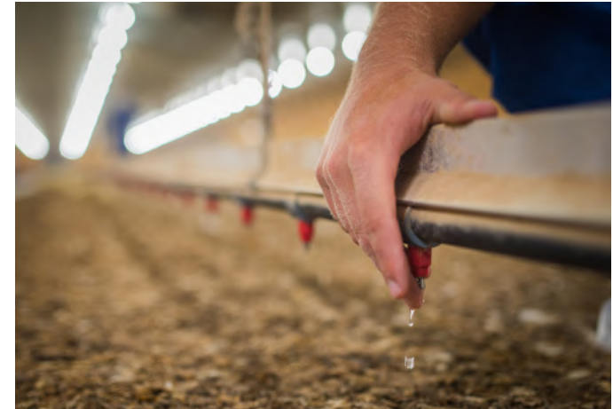
Prior to placement, check that all water lines and individual drinker nipples are operating correctly.
