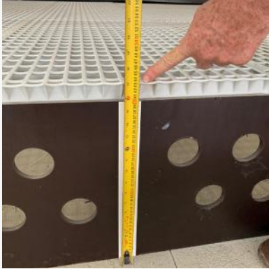
Slats should be 45 cm (18 in) high, measured from the top of the slats to the concrete floor.
