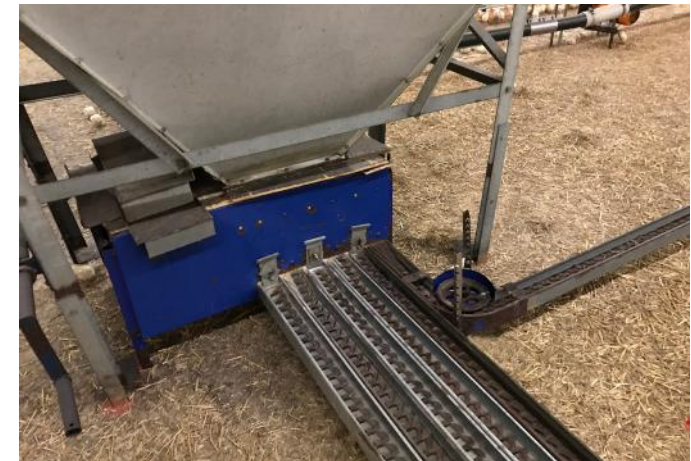
Run the feeding system and check that feed lines are level and secure.
