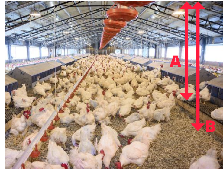
Airspeed uniformity is also affected by the height differential between the drop ceiling or roof and the scratch and slat areas. Prevent large differences in height between slat and the ceiling (A) compared with the scratch area and the ceiling (B).
