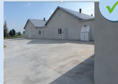
Surrounding concrete zone
