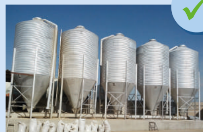
Silos in good conditions
