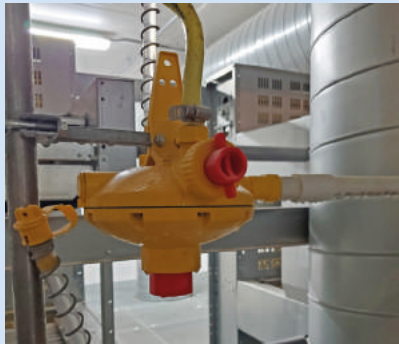
Flushing system (water regulator)
