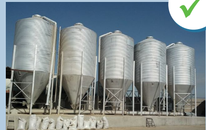
Silos in good conditions
