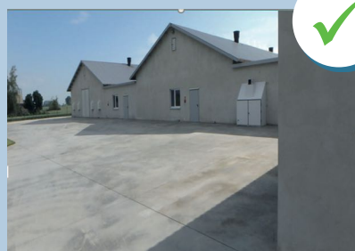
Surrounding concrete zone
