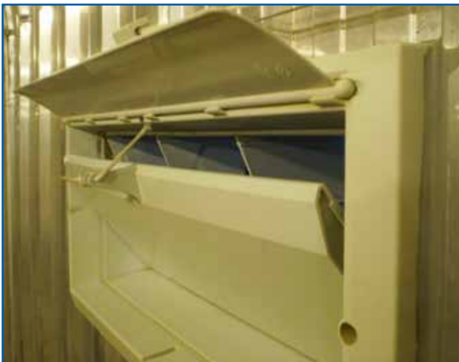
Figure 109: Example of a good-quality air inlet.
