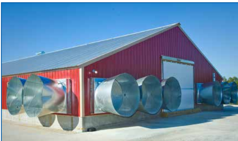
Figure 112: Example of a typical tunnel-ventilated house.
