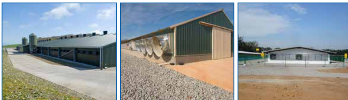
Figure 8: Houses with a low biosecurity risk showing concrete areas and no vegetation around the immediate perimeter of the house.
