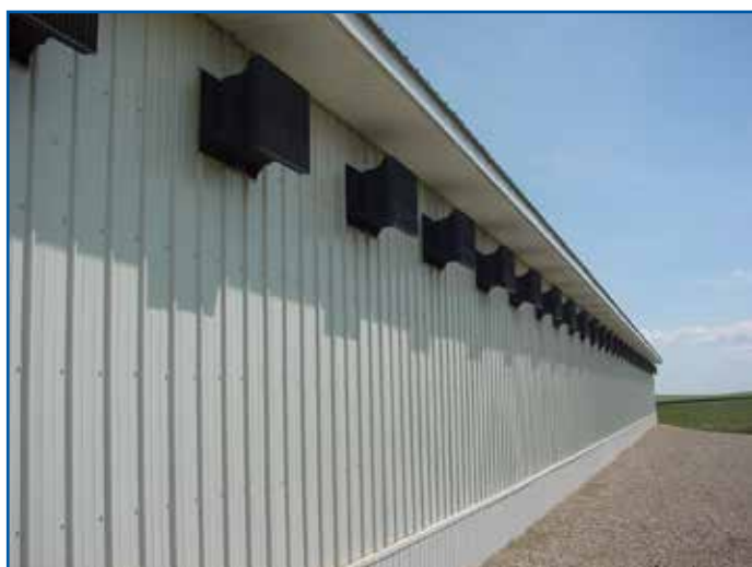
Figure 119: Example of a light baffle fitted to a cross ventilation inlet.
