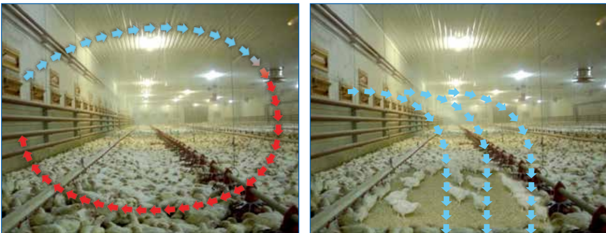
Figure 108: Illustration of air flow into the house. The picture on the left shows a correct fast air flow during minimum ventilation. The picture on the right shows an incorrect slow air flow during minimum ventilation.
