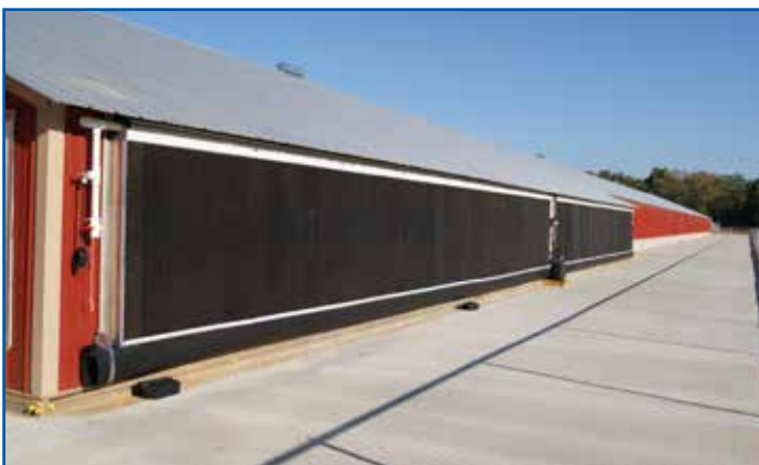
Figure 116: Example of a cooling pad.
