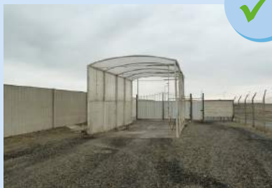
Disinfection tunnel for vehicles
